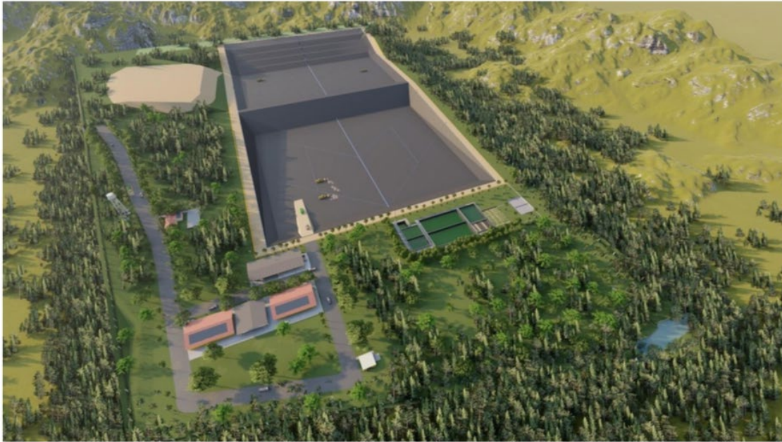
Figure 01. Aerial Perspective of a Category III SLF, highlighting the Emplacement Cell, Leachate Treatment Facility, and Total Solid Waste Management Facilities.
